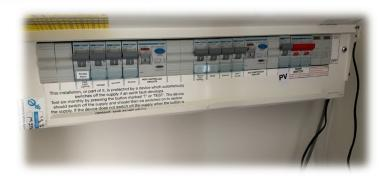
A High Integrity consumer unit will also future proof the installation should an EV charge point be required.
